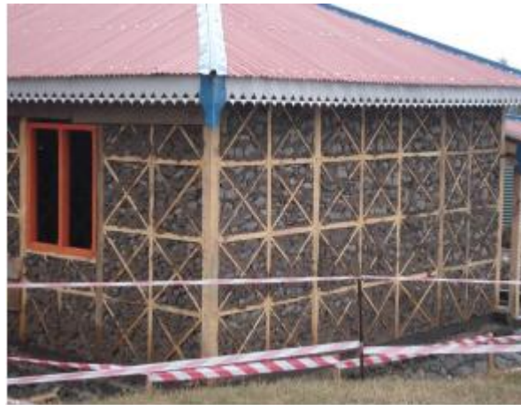
Figure 4: Dhajji Structures with mud masonry infill in Union Council Pashto, Battagram
